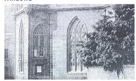
Existing windows are in a mixture of conditions with in some cases entire casements having fallen inwards. Large areas of leaded glass have been broken and sagging is an issue across most windows. Focusing on the larger buttress windows as main examples it is clear upon close inspection the windows have been altered and adapted from sash and case at some point.
