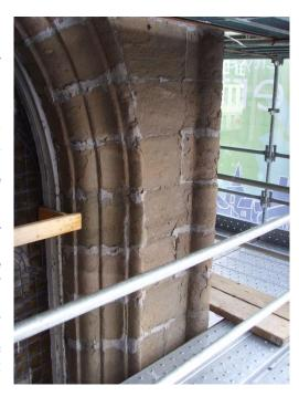
The weathering and cement damage effect to the stone has eroded the drove work finish and despite still having clear coursing has created a more rustic effect to the building. Internally it is not proposed to replicate the droved finish on any new stone with the exception of the piers at the new entrances. Externally it was decided that to try and replicate the droving across the building would be inappropriate
